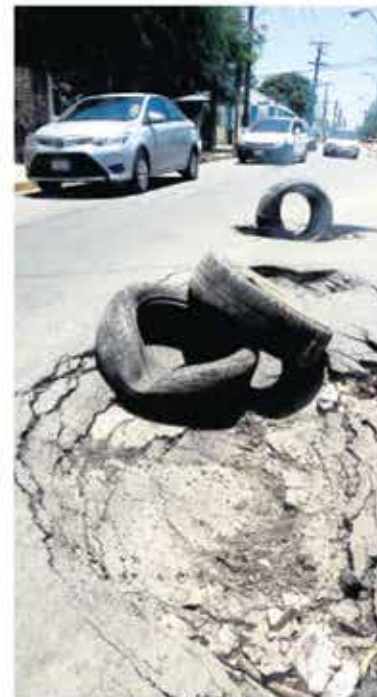
Sections of North Street, Kingston, between East Street and Rum Lane, have started to collapse only a few months after major pipe laying and repairs to the road.
