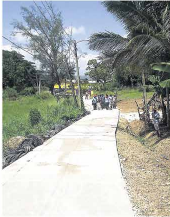
The new paved road leading to Bermaddy Primary School in St Catherine.
